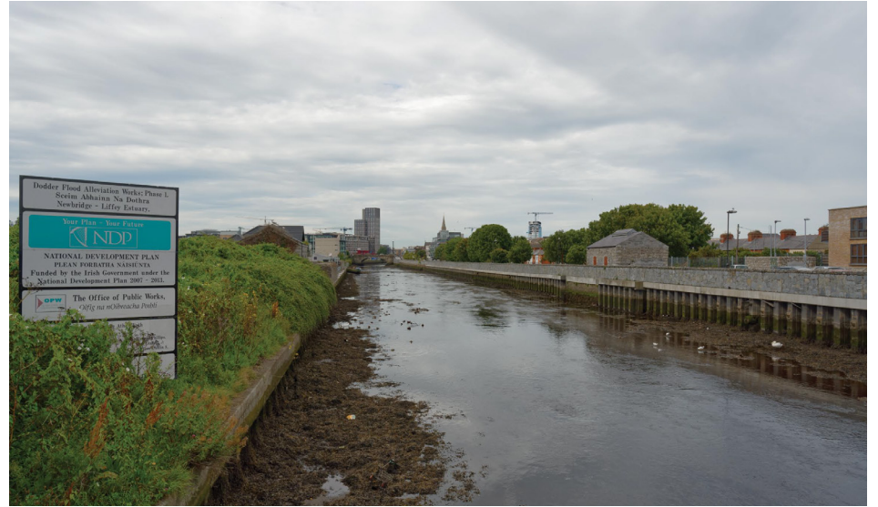
Figure 10.3: View 25 from Bath Road along River Dodder - existing situation
